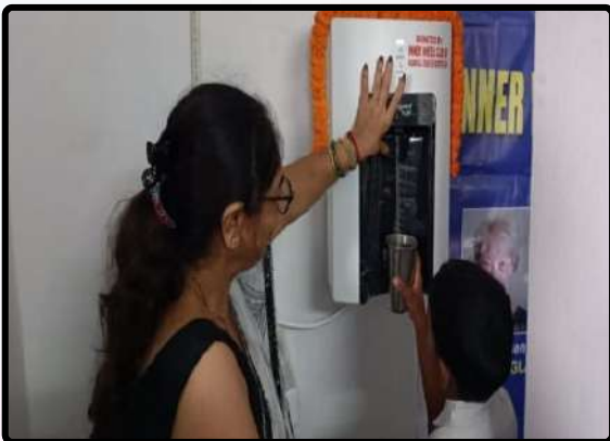
INSTALLATION OF WATER PURIFIER AT OUR ADOPTED SCHOOL Amount Spent - Rs.6000
